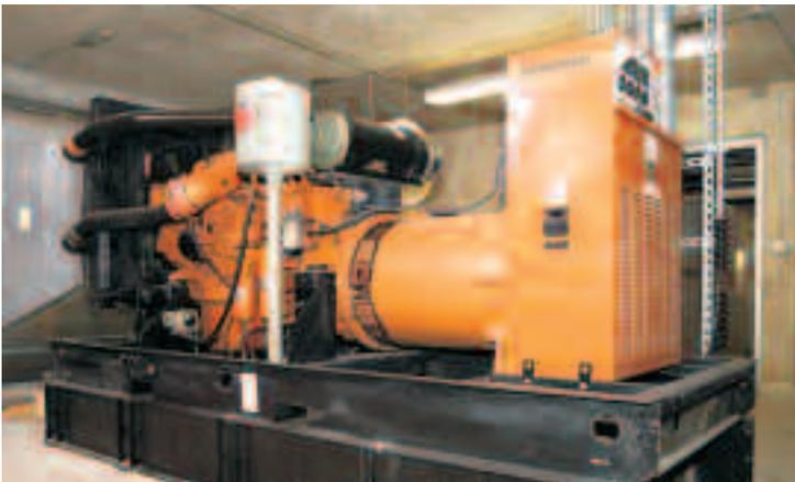
**3** Redundant refrigeration systems provide continuous fail-safe cooling in the event one unit stops working. During extended power outages we have you covered, our 13.3 liter diesel-powered electric generator with 2,000 gallon fuel storage capacity provides over two weeks of continuous electrical power to our redundant cooling systems.
